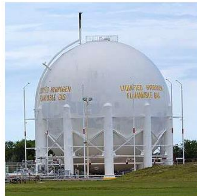
Liquid hydrogen storage tank at Kennedy Space Center was used to fuel the space shuttle. (TomFawls 2013, creative Commons 3.0)
